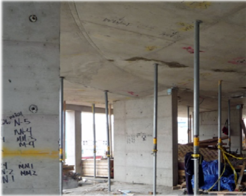
Figure 17: View of transition from 9" slab to 18.5" slab
