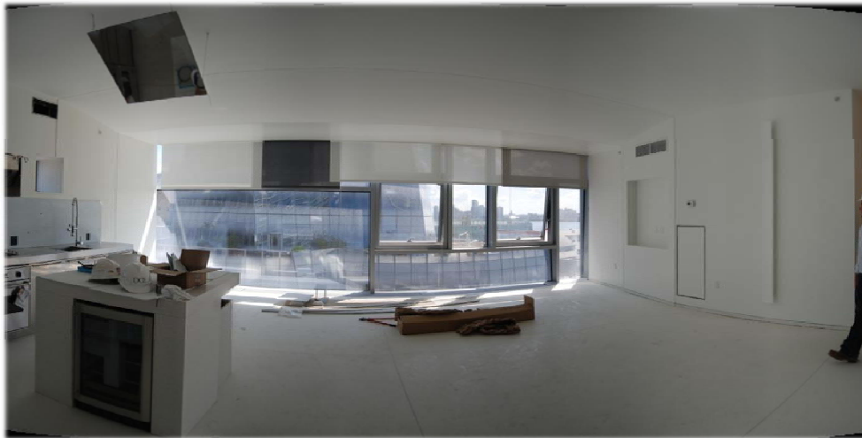
Figure 54: Interior of residential unit showing current shading devices
