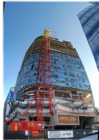
Figure 61: View from street level
