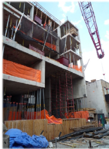
Figure 18: Cantilevered slab as part of balcony system
