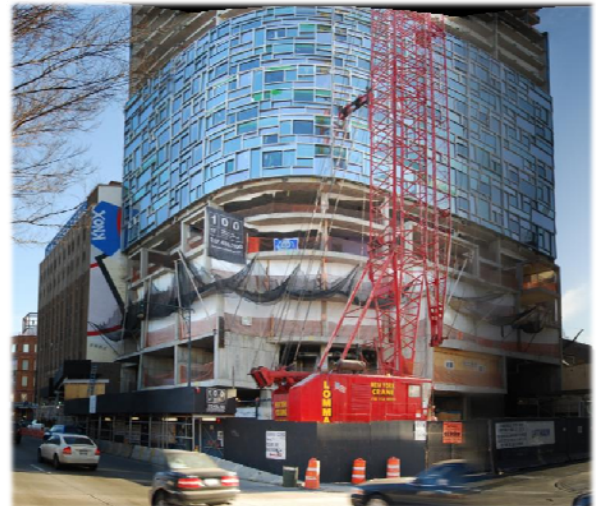
Figure 57: View of panelized facade from south-west corner
