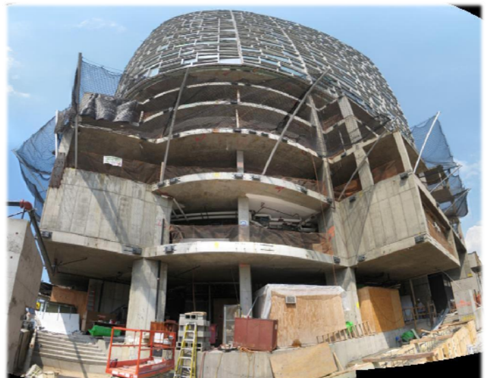
Figure 12: Photo showing portion of cantilevered balcony system
