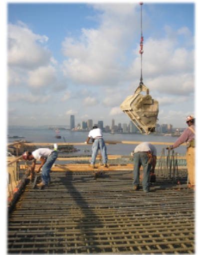
Figure 19: Heavily-reinforced 19th floor transfer slab
